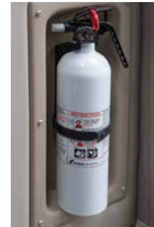
Typical Class B-C fire extinguisher
